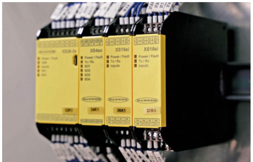
The Banner SC26 safety controllers process all safety-related signals
